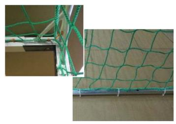
b) Fix ends of upper and lower tensioning rope at the mounted ring nuts. Cut off protruding rope ends (see bottom picture).
