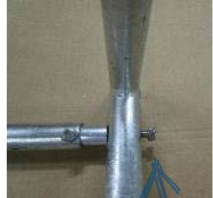
1. nut outside flush with screw
