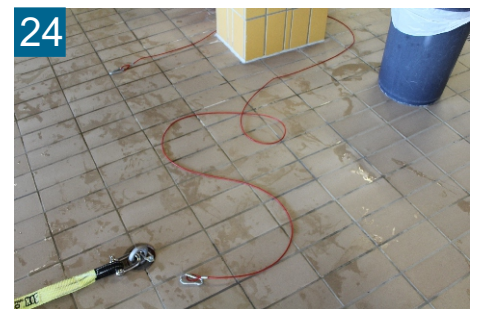
24 Put safety rope in the mount
