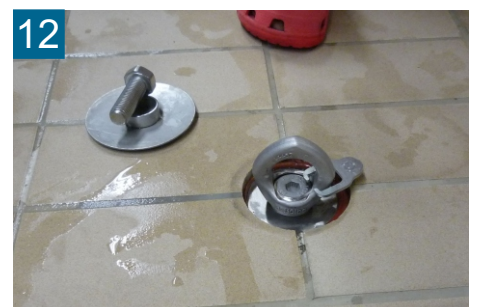
12 Tighten fixing screw manually as deep as possible loosen allen key
