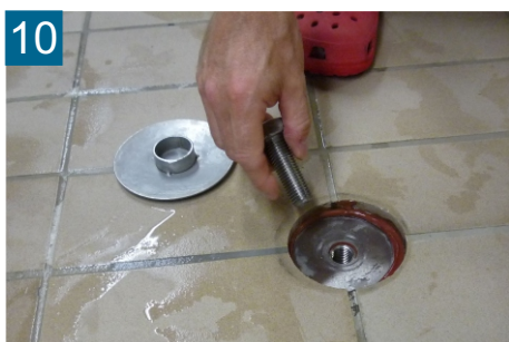
10 Remove protection screw
