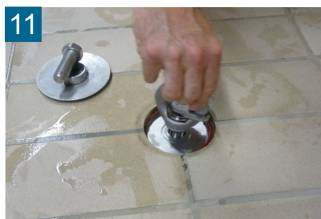
11 Fix allen key, turn the fixing screw
