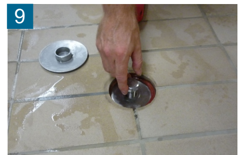
9 Unscrew protection screw
