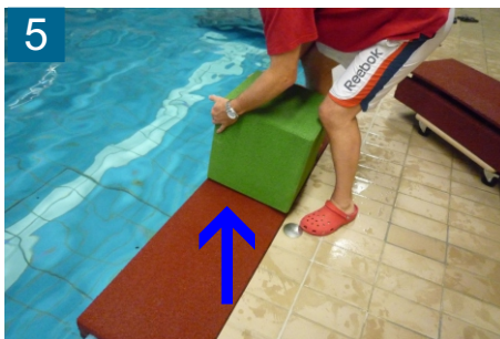
5 Place EPDM cube precisely in the middle
