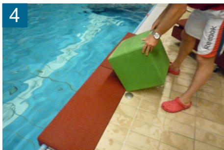
4 Place EPDM cube precisely in the middle
